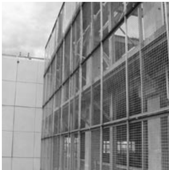
Figure 18 View of perimeter screens from the outside
