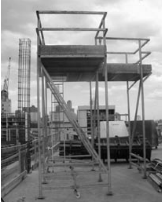
Figure 5 Mobile fabricated column formwork platform
