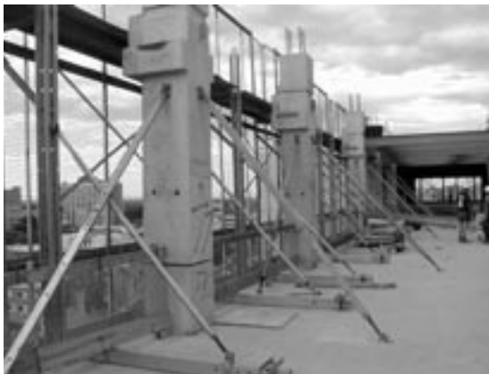
Figure 7 Perimeter screens secured by props
