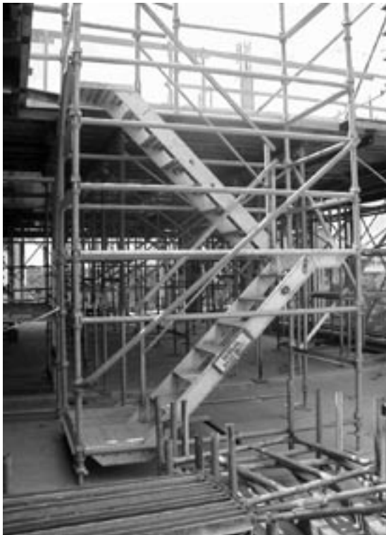
Figure 19 Access to form deck
