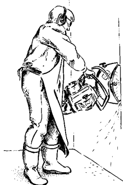
Using a concrete saw requires the application of high force and sustained awkward postures of the back and neck.
