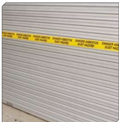
Figure 3: Barrier formed using tape (appropriate for small non-friable removal jobs or as part of system using other barriers such as hoarding).
