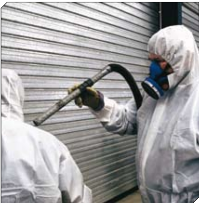
Figure 7: 'Buddy' cleaning – decontaminating colleagues with a HEPA vacuum cleaner.
