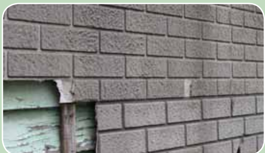
Asbestos cement 'brick' cladding
