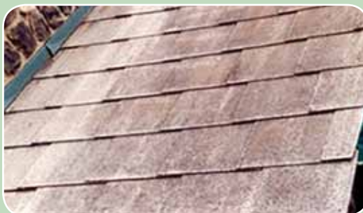
Asbestos cement shingles
