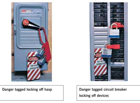
Figure 1: Locking off methods incorporating danger tags
